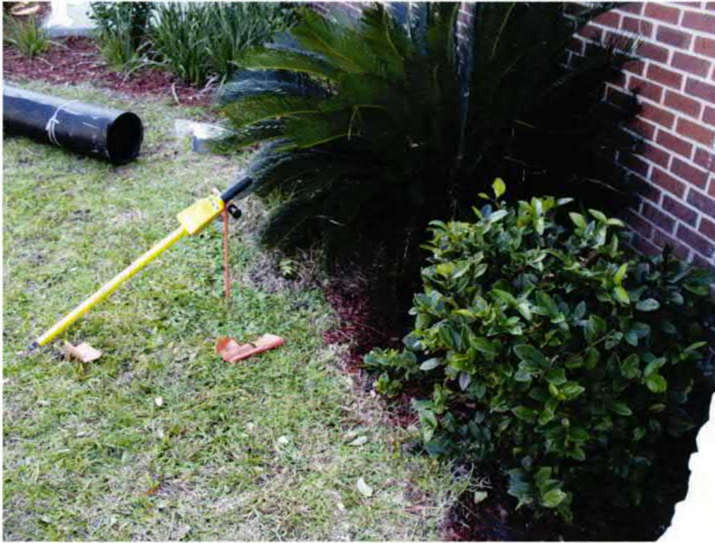
Picture 1: Location of UST 566Dahlia.
